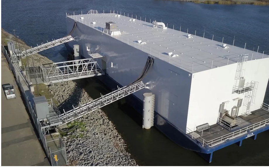
Fig. 2. The first water-borne datacenter in Stockton, California claims to achieve a PUE of 1.15, using a raw water flow of approximately 4,500 gallons per minute (GPM), with a maximum capacity of up to 12,000 GPM from its eight pumps [59].
